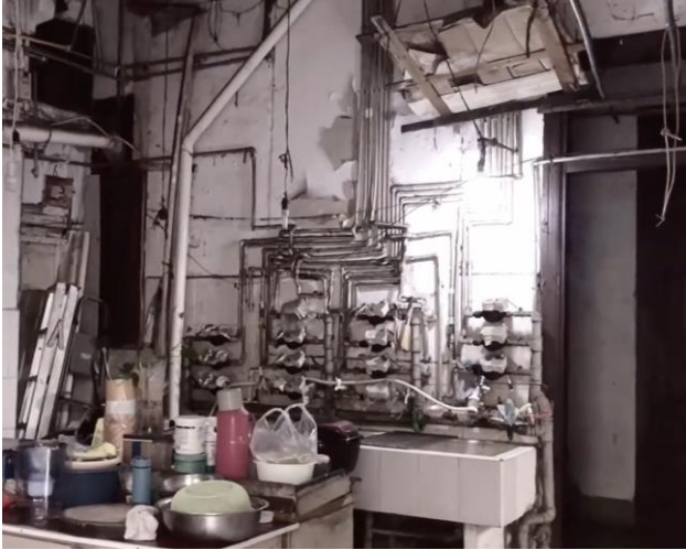
Fig.15: More than a dozen water meters belonging to several families in the same stove, Haiyan Wang, 2023
